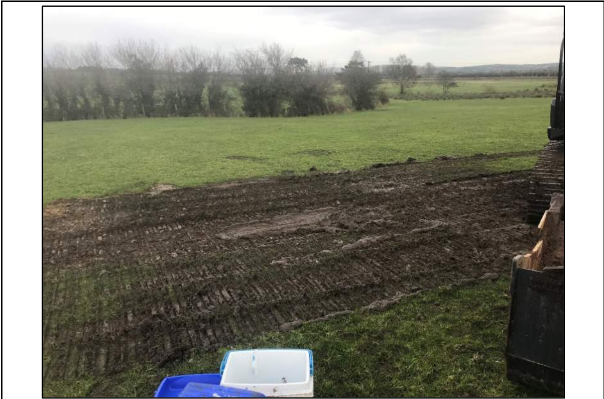
Tracks around TP2 excavation
