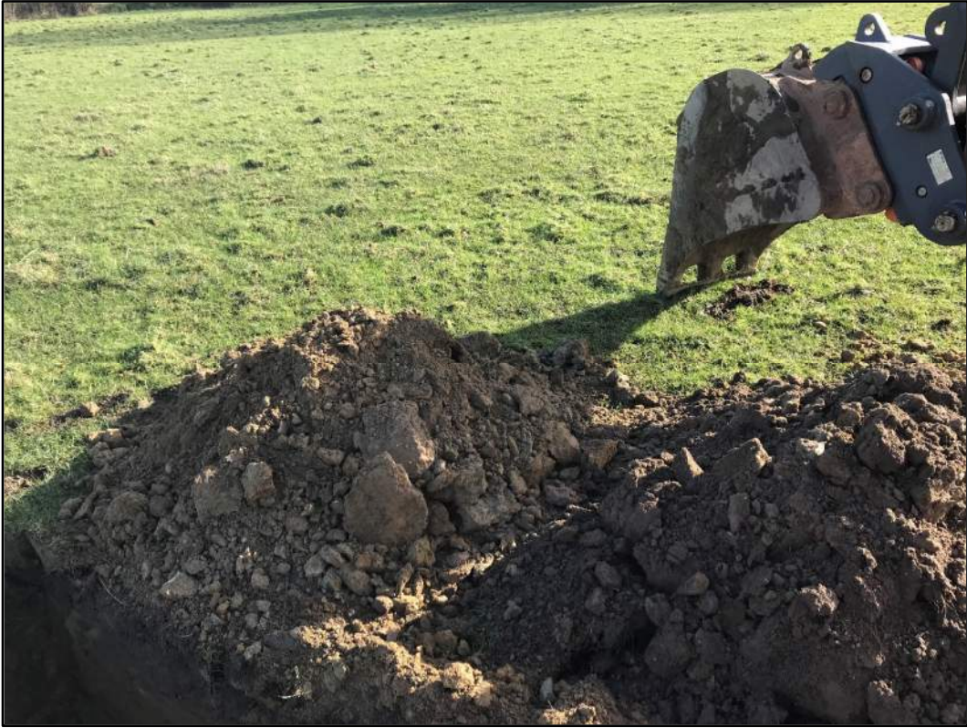
Material removed from TP8 excavation
